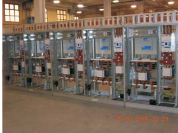
Tamarindo – 30 Pumps at 450HP each
